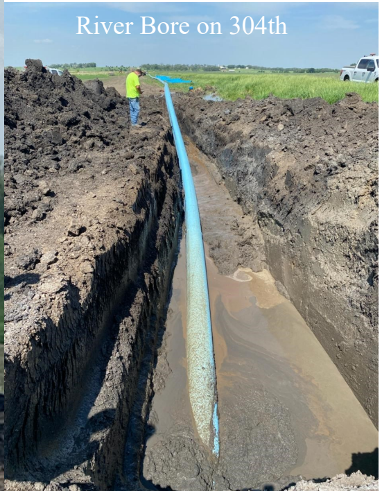
304th Pipe Ready to Install
